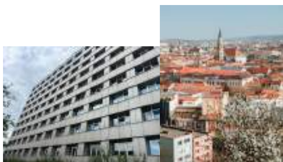
Fig. Cluj (Romania) - Renovation of students accommodations
