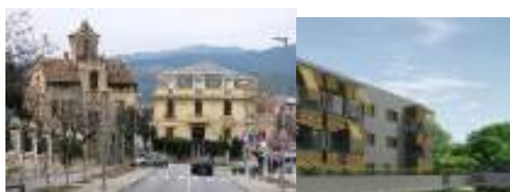
Fig. La Garriga (Spain) - Private apartment blocks
