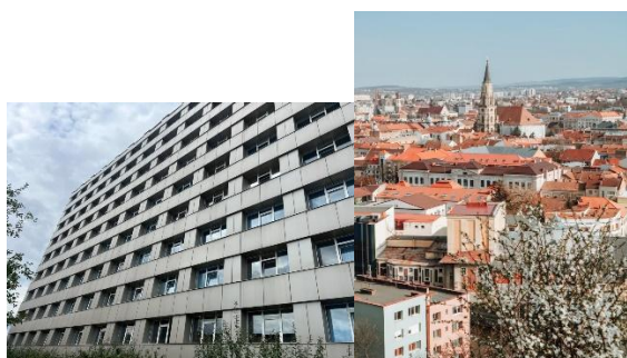
Fig. Cluj (Romania) - Renovation of students accommodations
